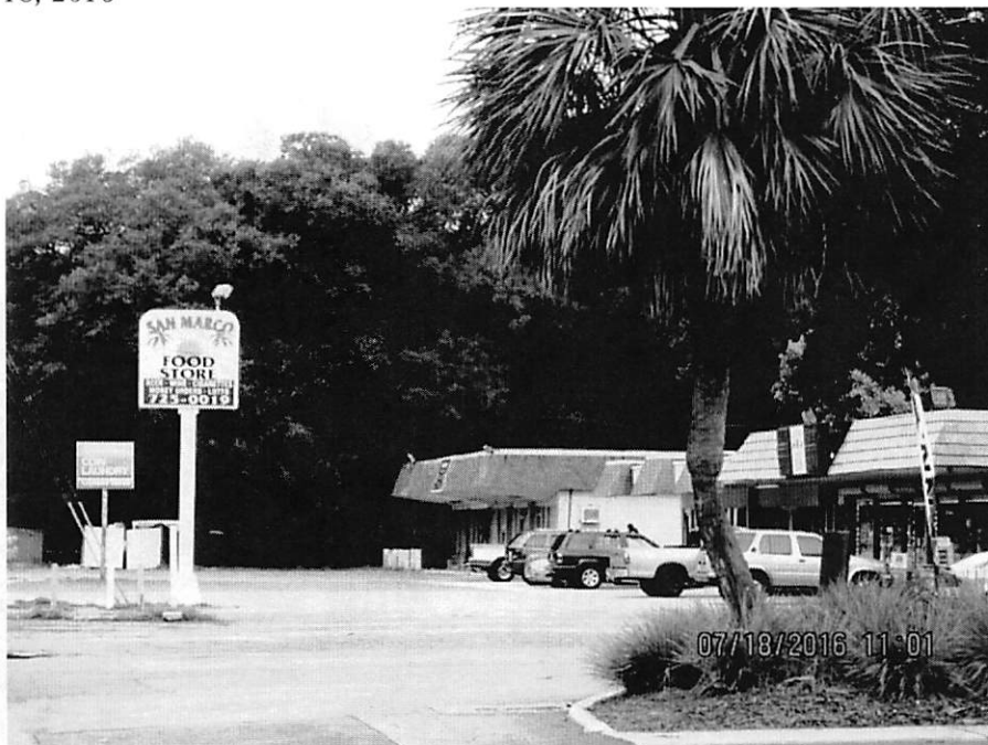
Existing commercial signs to the west, with similar encroachments
